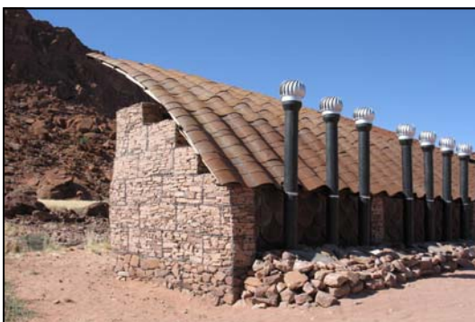
The new visitor centre at Twyfelfontein is installed with dry toilets. Note the air escape vents. © N.Maritz
