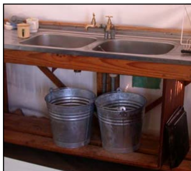
Buckets under the kitchen sink allows you more options in deciding where the wastewater should go—relatively clean water can be used to water the garden. © N.Maritz
