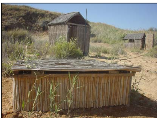
This reed walled flush loo drains into a well concealed septic tank © P.Tarr
