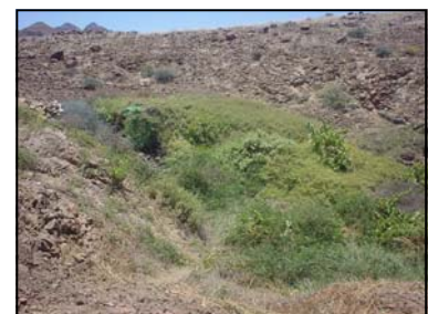
Leaking pipes often go undetected, even though this patch of green vegetation near the water tank is a clue to a leak © P.Tarr
